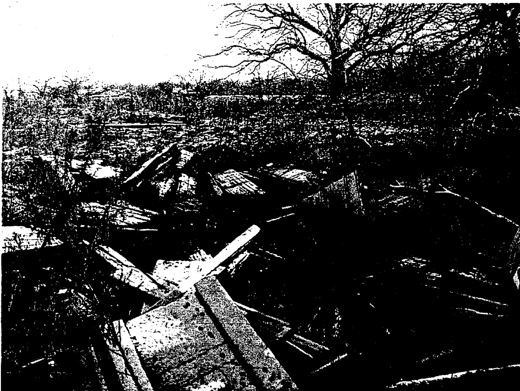
Date: December 1, 2004 Time: 10:25 Direction: W-SW Photo by: S. Townsend Exposure #: 006 Comments: Demolition debris from grain elevator in tributary to Sugar Creek in Dump Area C
